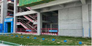
▲ Sound insulation and noise reduction screen is erected for rebar processing
