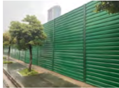
Sound-proof enclosure boards at Haikou CR Center Crossing
