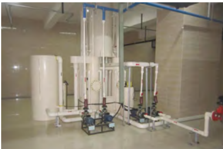
Reclaimed water treatment equipment
