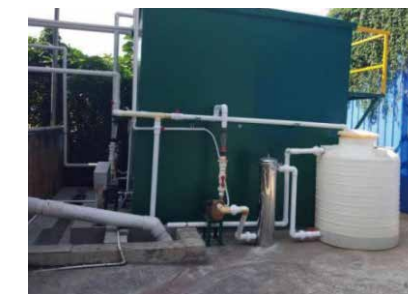
New MBR membrane biochemical pool and wastewater testing equipment
