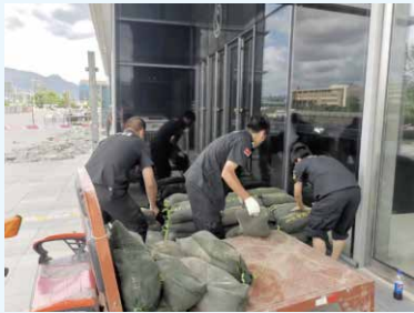
Deploy flood-proof sandbags in advance in operation projects
