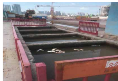
Wastewater three-stage filtration
