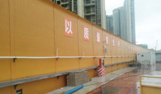
Sound-proof enclosure boards of Shenzhen Runxi Phase I
