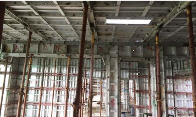
Aluminium mould construction of the Hainan Shimei Bay Project
